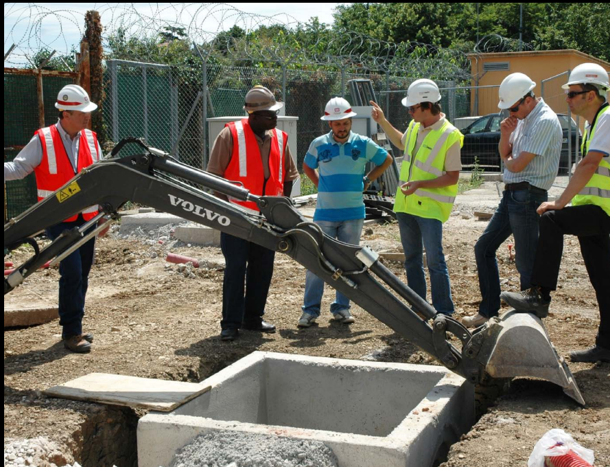
Left to Right: John Curtis and Howard Mosley visit construction sites in Longare, Italy. Not pictured: Mark Nedzbal, Rob Eldred, Michael Pfaff, Laura Berto, James Alexander, James McMullen – Livorno Office and John Thomas – Aviano Office
