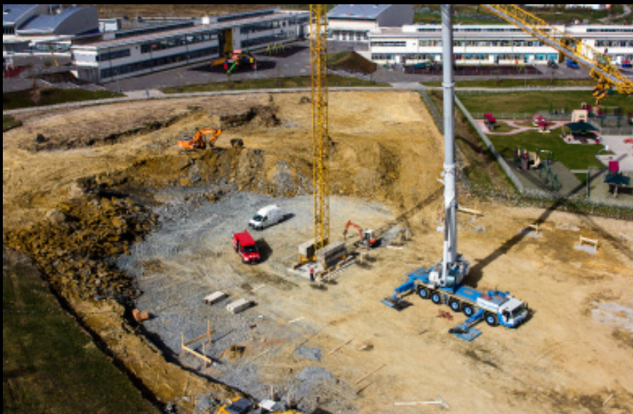
Site preparation continues for the future Netzaberg Chapel at U.S. Army Garrison Bavaria in Germany, the final project under Efficient Basing Grafenwöhr. The 600-person facility will include an activity center, kitchen, religious education areas, resource center, sacristy room and administrative spaces. (Courtesy of Andrea Hoesl/USAG Bavaria, DPW)
